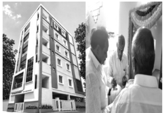
View of LDR Bhawan (NFTE BSNL) at hyderabad built by district union
